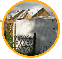
Rainwater is used for bathrooms, toilets and gardens
